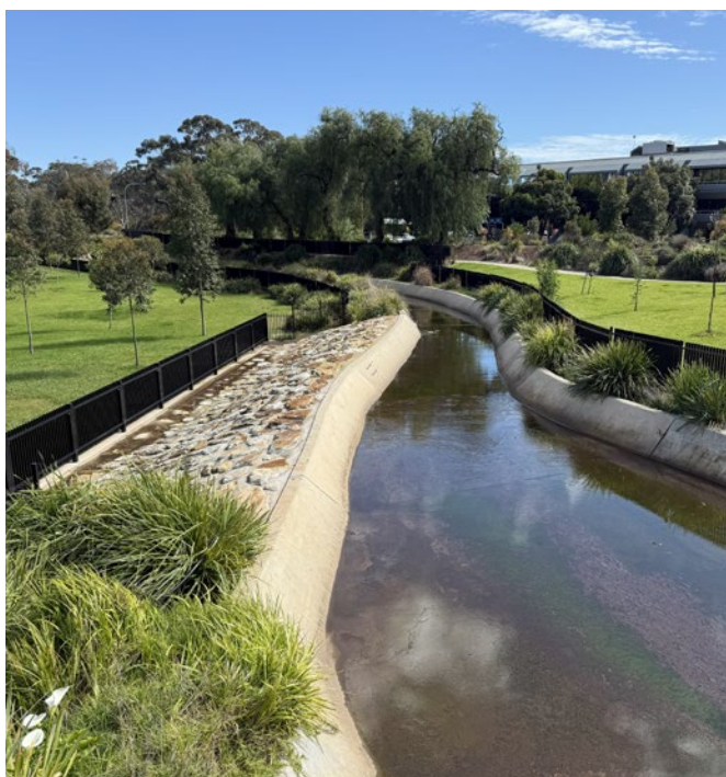
Glenside concrete swale
