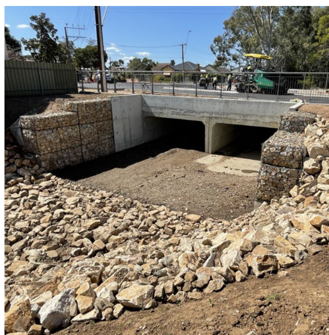
Bridge Upgrade - After
