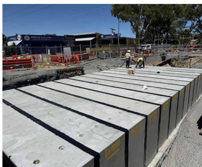
Lower Brown Hill Creek Upgrades - culvert installation
